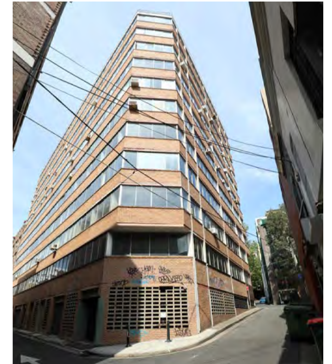
View 9. Looking south along Terry Street
