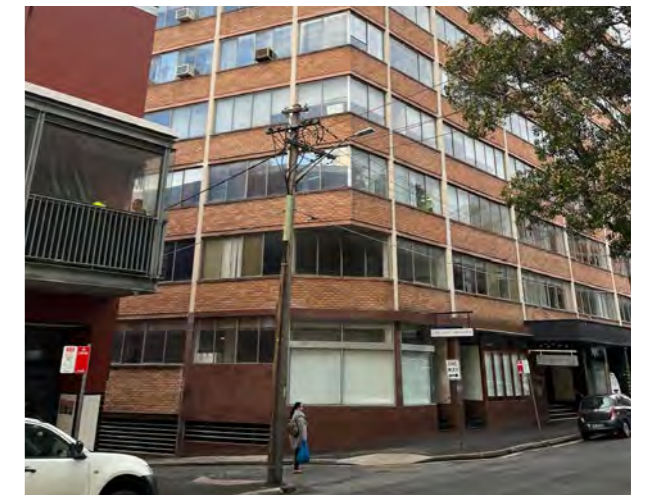
View 6. Looking east along Kippax Street
