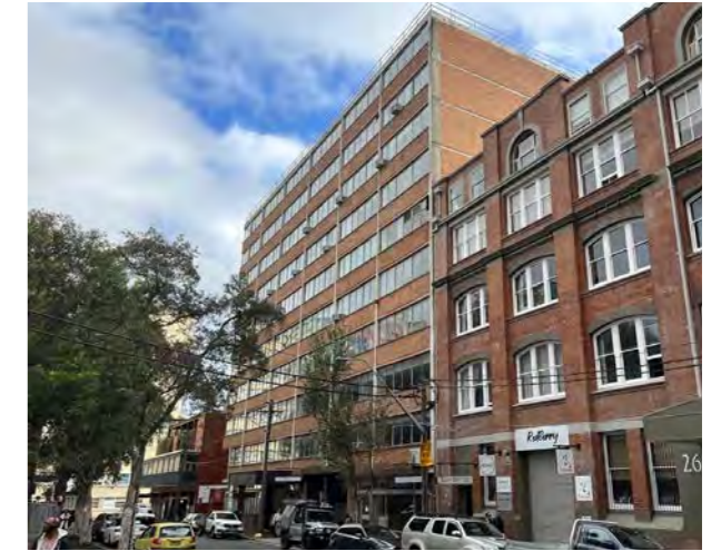
View 3. Looking north west at corner of Holt and Kippax Street
