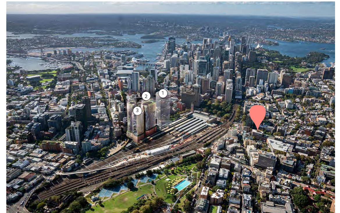
* Aerial view looking north west
